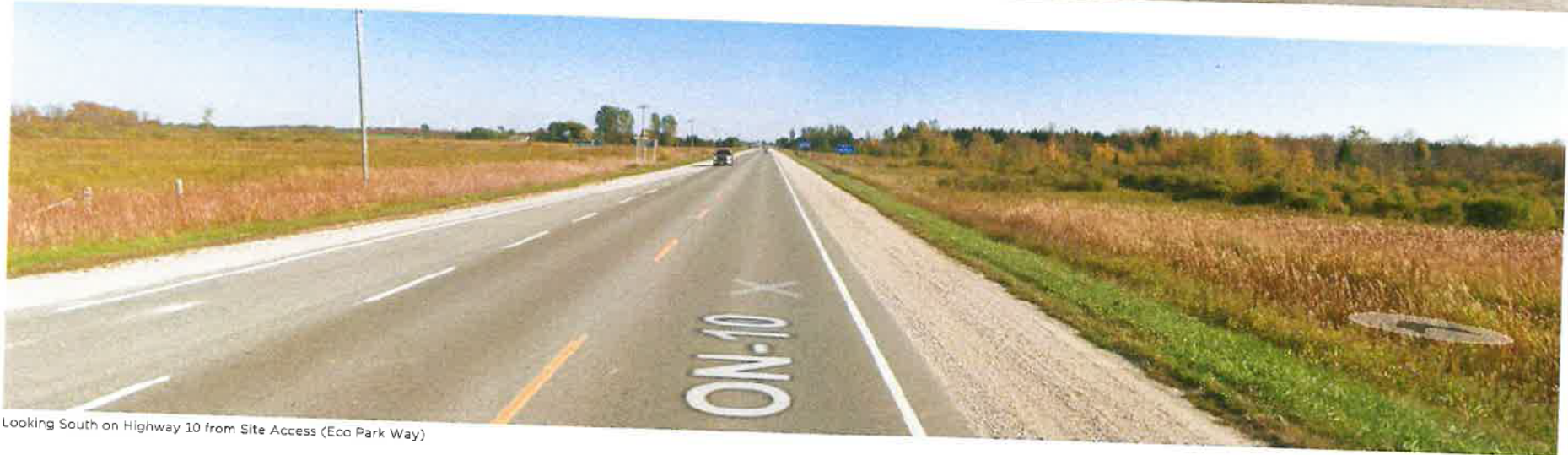
Looking North on Highway 10 from Site Access (Eco Park Way)
